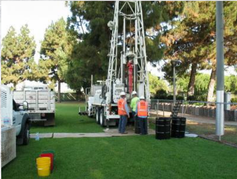
GMW-65 Drilling Set Up
