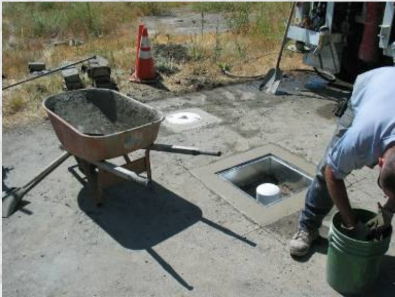
GW-16 Surface Completion
